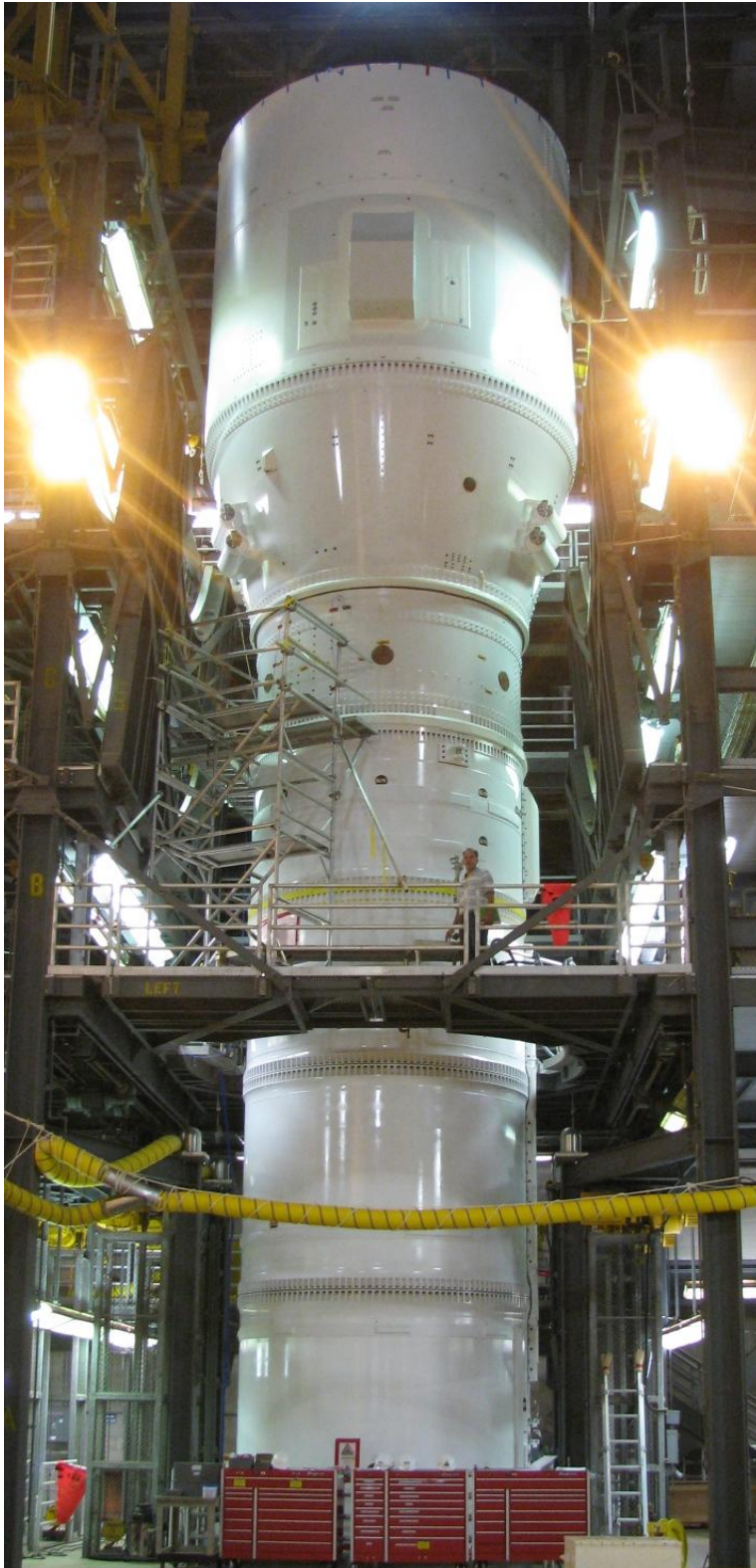
Figure 3. Stack 1 test configuration
