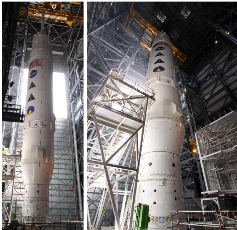
Figure 10. Upper Stage of Ares I-X Vehicle extends above the facility access platforms.
