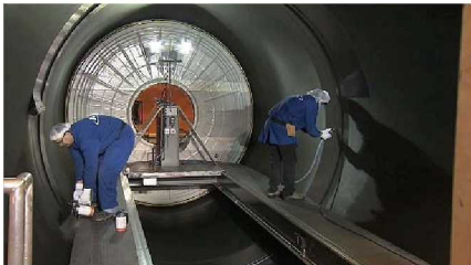
Asbestos-free insulation/liner. Thickness changes will be modified during Development Motor testing
