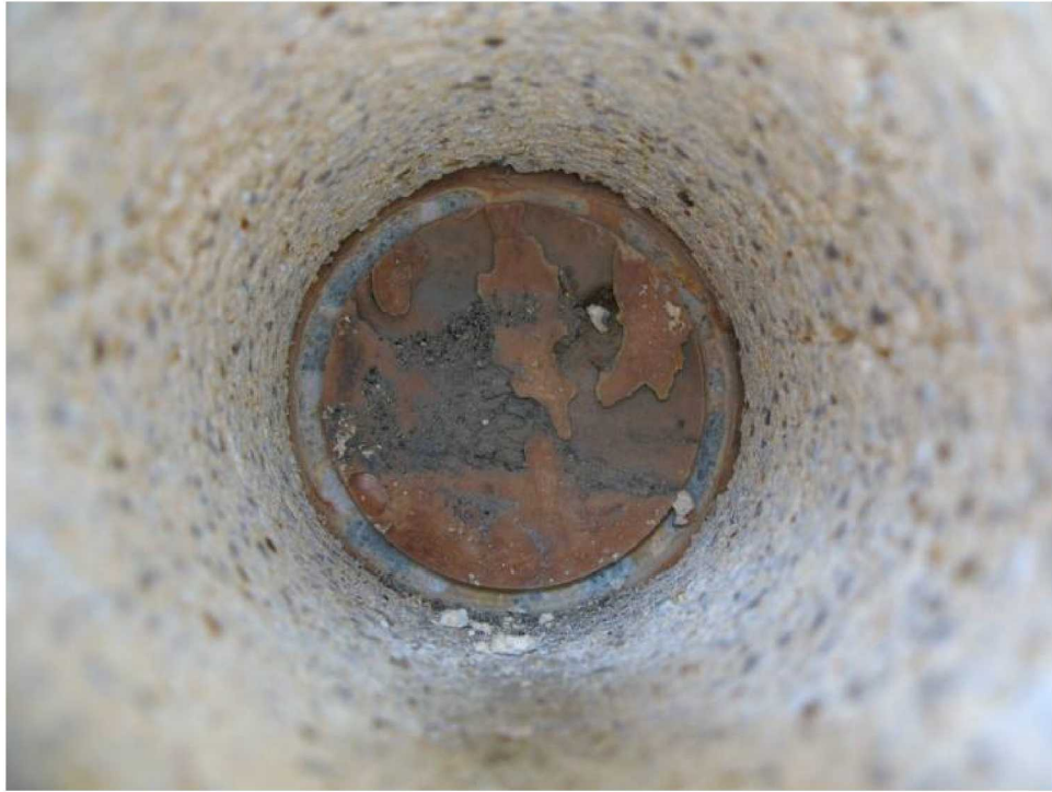
Figure 41. Core 11W –inside the brick after the core was removed
