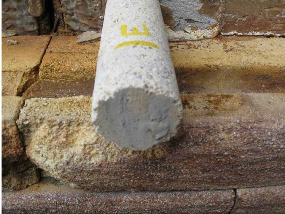
Figure 9. Core 1E – inner surface of core removed during core drilling
