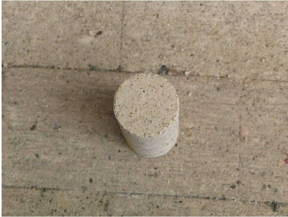
Figure 31. Core 6W – inner surface of core removed during core drilling
