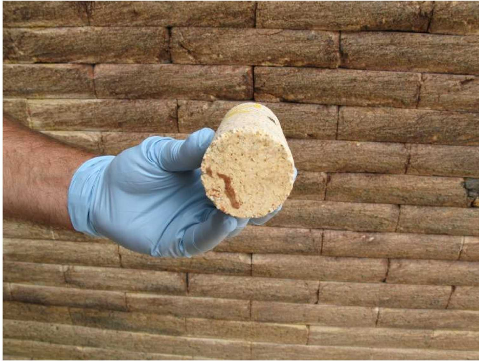
Figure 33. Core 7W – inner surface of core removed during core drilling
