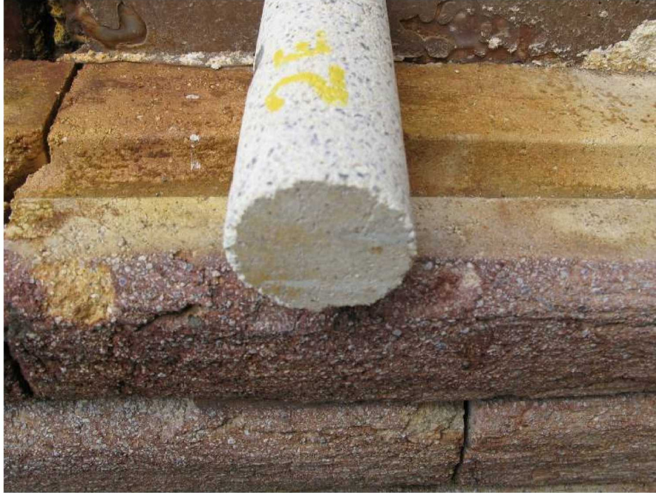
Figure 11. Core 2E – inner surface of core removed during core drilling
