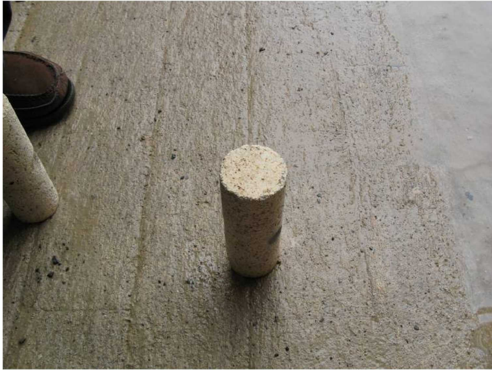
Figure 27. Core 4W – inner surface of core removed during core drilling
