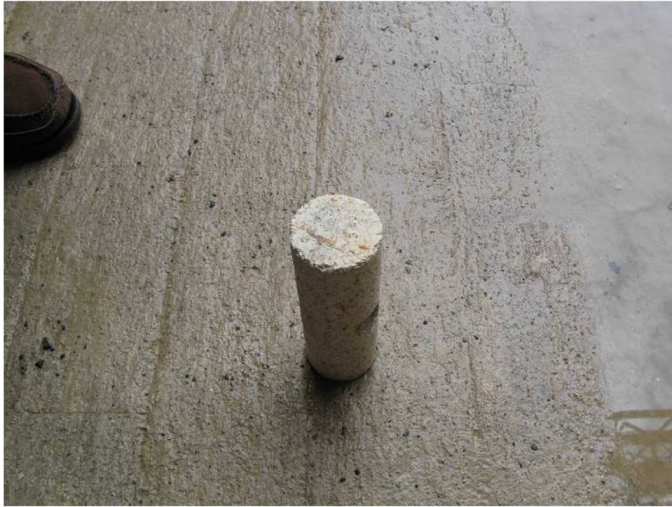
Figure 29. Core 5W – inner surface of core removed during core drilling
