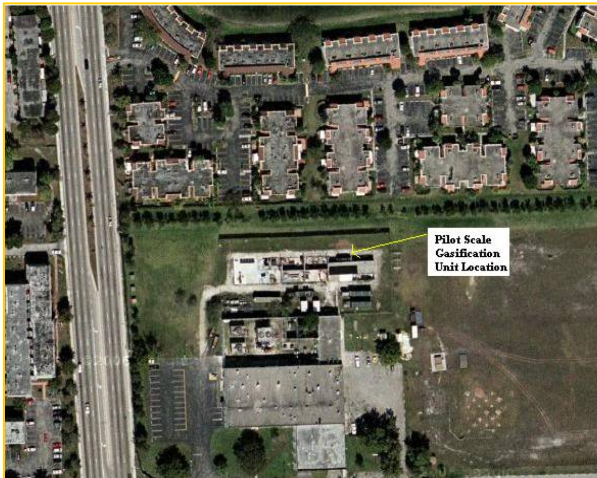
Figure 4. FIU's gasification unit location.
