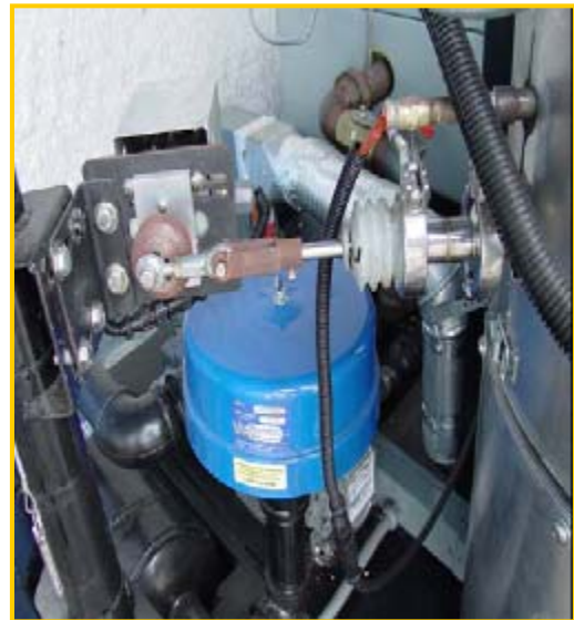
Figure 8. Char Air Tree (Left) and Grate Shaker (Right).
