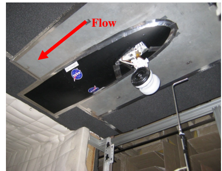
Figure 3. Installation of pitot static probe for flow speed measurements.
