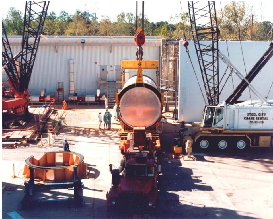
Figure 13. A variety of cranes will be used to move IVGVT hardware from transportation facilities to Test Stand 4550.
