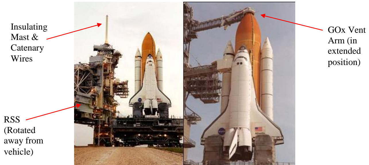
Figure 6.0-1. Pad 39B Lightning Protection
