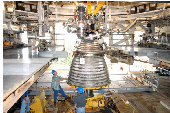
Figure 6. Powerpack 1A during test stand installation at Stennis Space Center.
