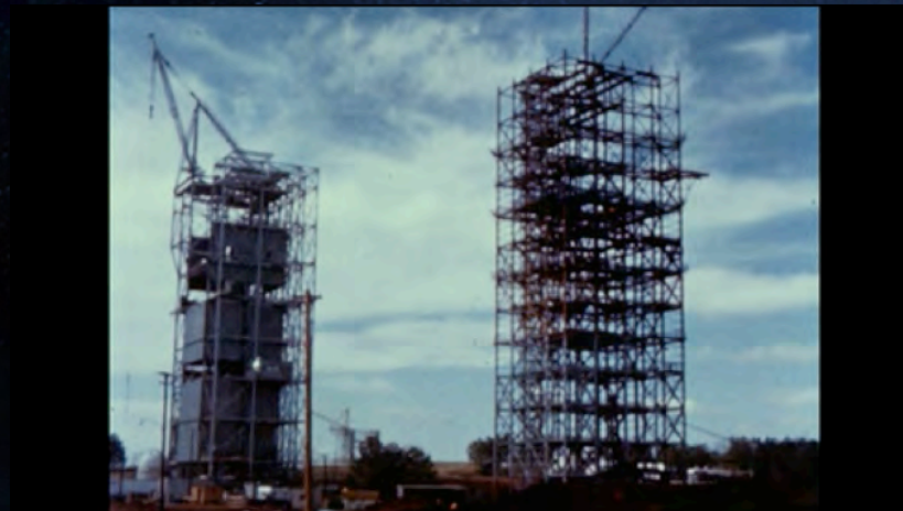
Dynamic Test Stand Renovations Marshall Space Flight Center, AL
