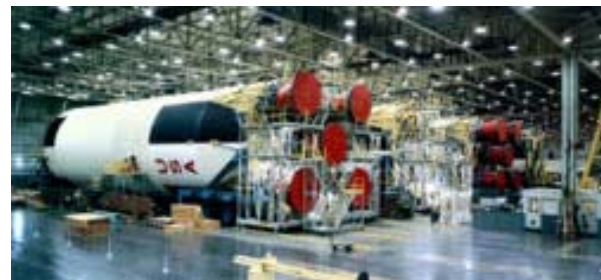
construction at MAF in 1968.
