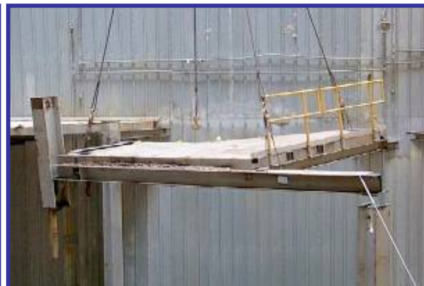
A section of the platform being removed
