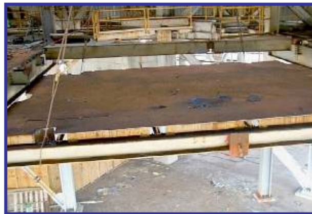
Lowering of the crosswalk to facilitate platform removal
