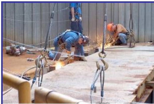
Workers cutting a section of the platform prior to removal
