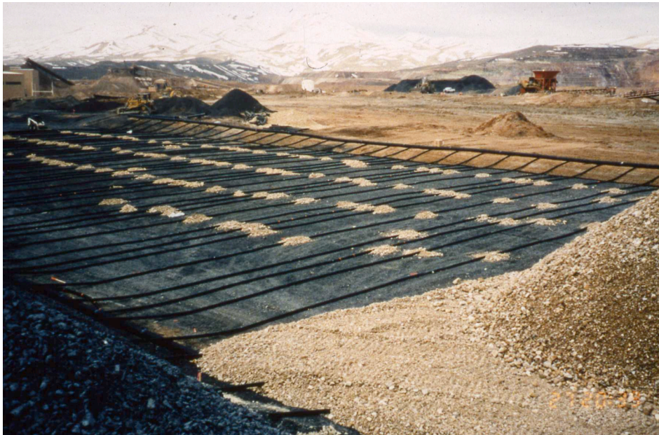
Figure 3: Active ventilation by forced air ~ 1995, The Quebrada Blanca Cu Leach.
