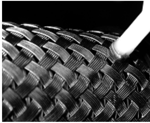
FIGURE 2. Probe orientation implemented to inspect for circumferential cracking in the flex hose convolute.
