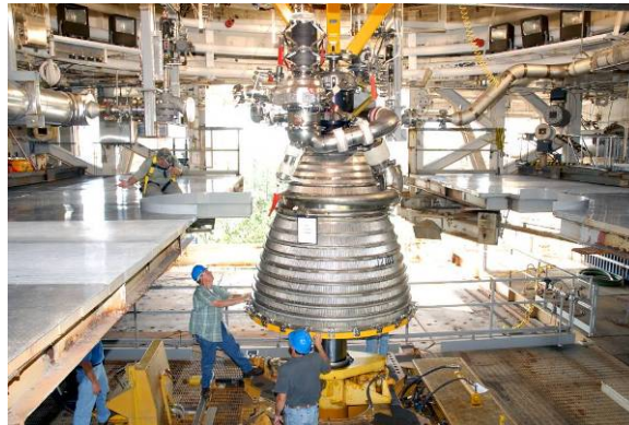
Figure 5. Powerpack 1A during test stand installation at Stennis Space Center.
