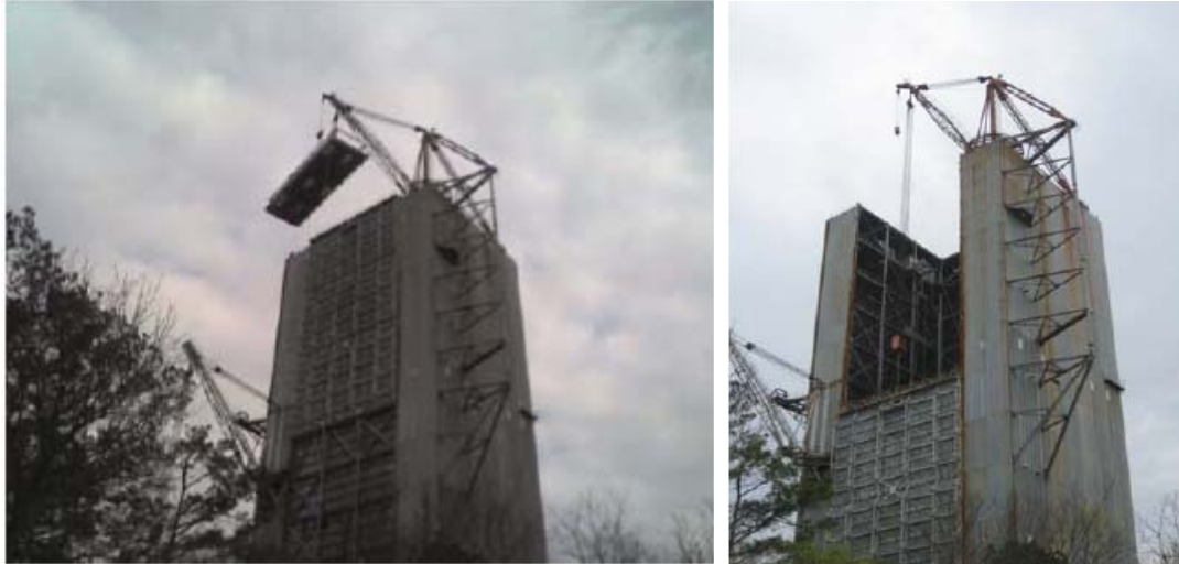
Figure 8. The side door was opened on Test Stand 4550 and the roof panels were removed for the first time in 29 years this past April.
