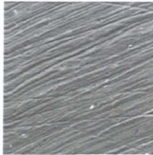
Removed remaining Koropon - sect 4A sanded 400 grit to breakthrough mostly no conductance
