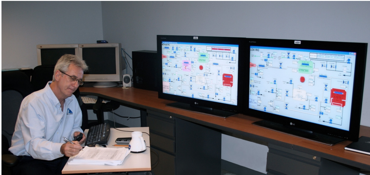
Figure 5. HMI Control System for operation of the PCFS test rigs
