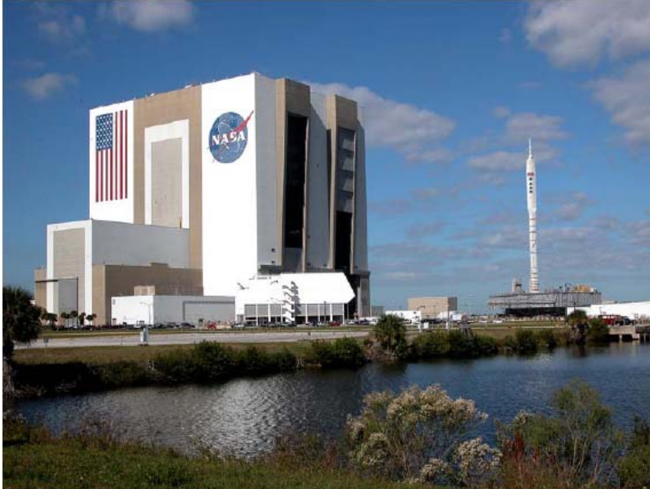
Figure 16. The VAB (left) will modify existing Shuttle handling hardware to stack Ares I-X.
