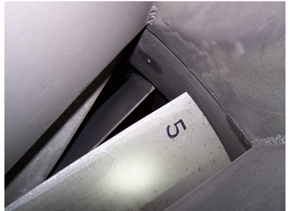
Probe Installation -Fan Interior
