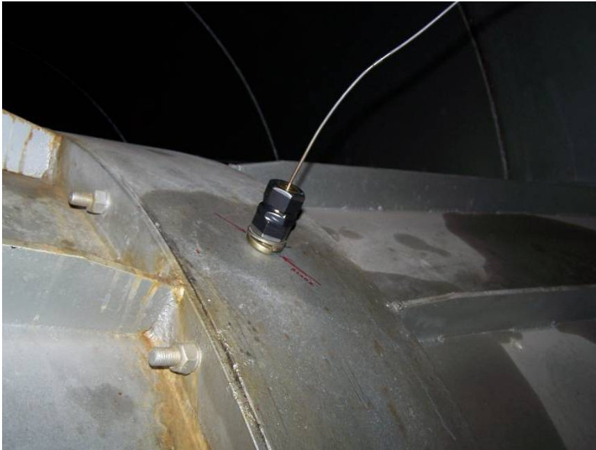
Probe Installation - Fan Exterior
