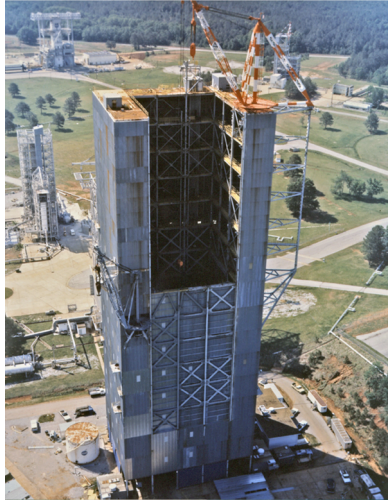
Fig. 15. TS 4550 is being modified for Ares I testing in 2011.
