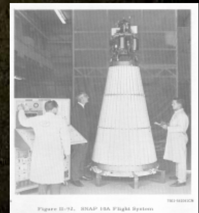
Figure D-92. SNAP 10A Flight System
