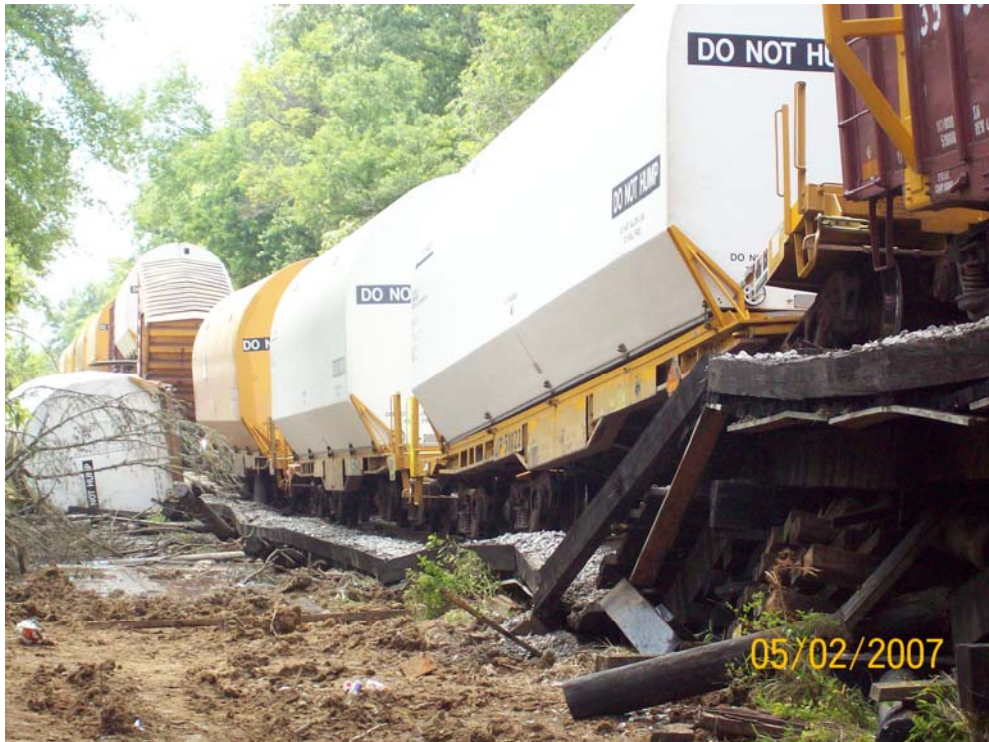
Figure 5. Segments On the Collapsed Trestle
