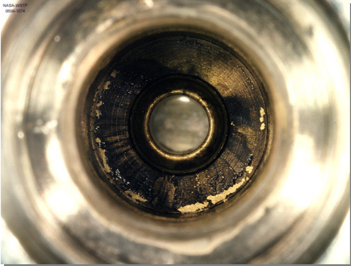
Tank Cylinder Valve
