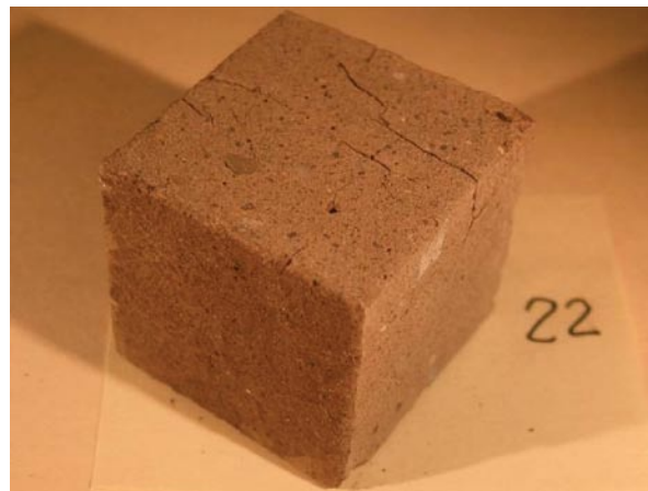
Figure 31. Photograph of cracking exhibited on the surface of sample 22, which was subjected to 80 cycles between RT ( \approx 21\text{ }^{\circ}\text{C} , or 70\text{ }^{\circ}\text{F} ) and -191\text{ }^{\circ}\text{C} ( -312\text{ }^{\circ}\text{F} ).
