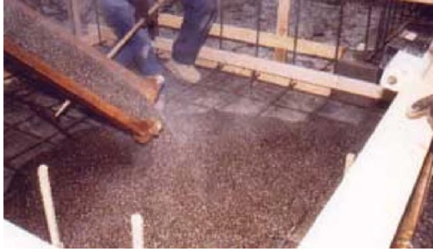
Figure 2. Pouring of Chempruf Sulfur Concrete in an industrial plant.
