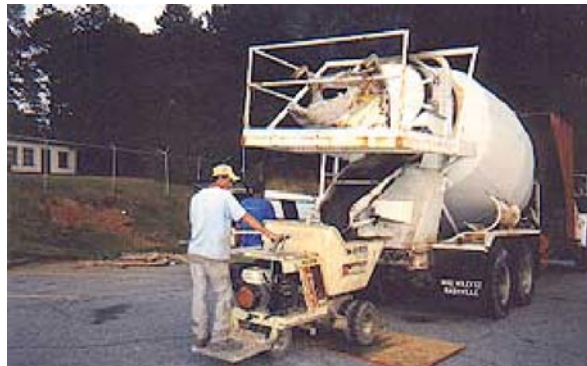
Figure 1. Eight-cubic-yard heater-mixer mobile production unit.
