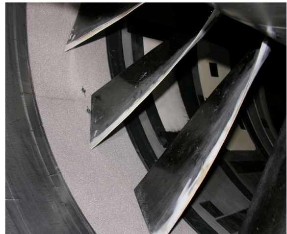
Figure 11. FML Spool Installed over Rotor.
