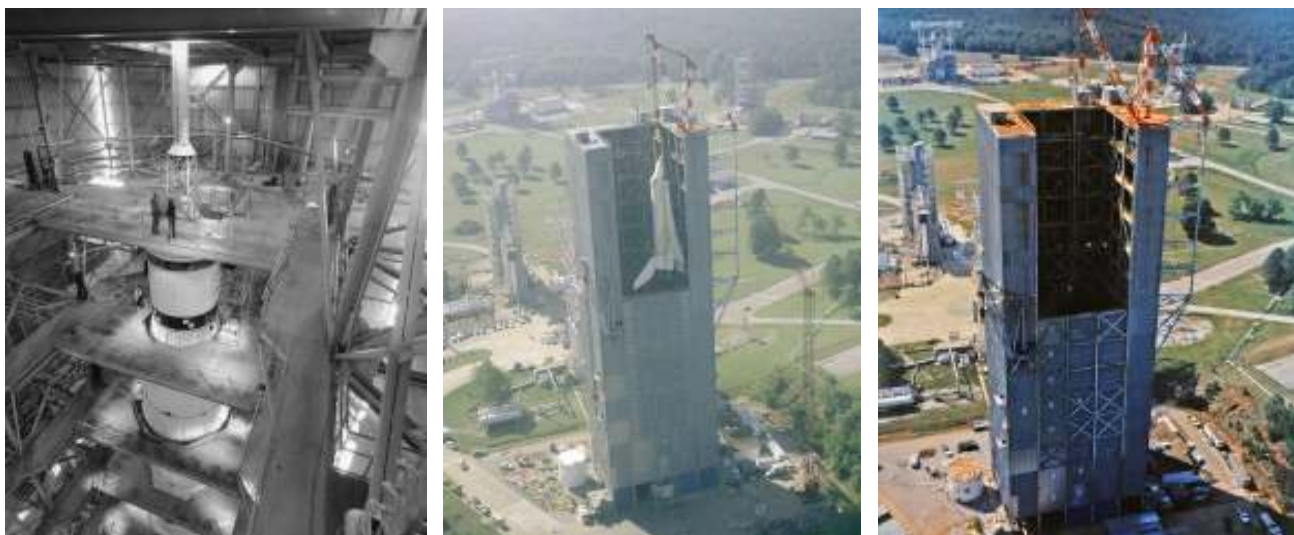
Figure 7. Photographs of the MSFC Dynamic Test Stand representing (from left to right) Saturn V testing, Space Shuttle dynamic testing, and prior to refurbishment for Ares I testing.
