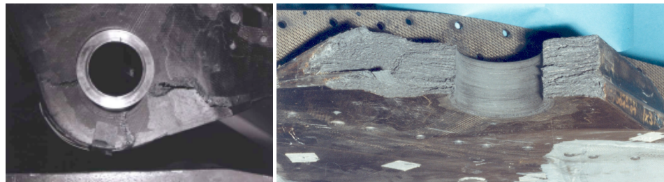
Figure 20. X2/2 Test Specimen – Observed Failure.
