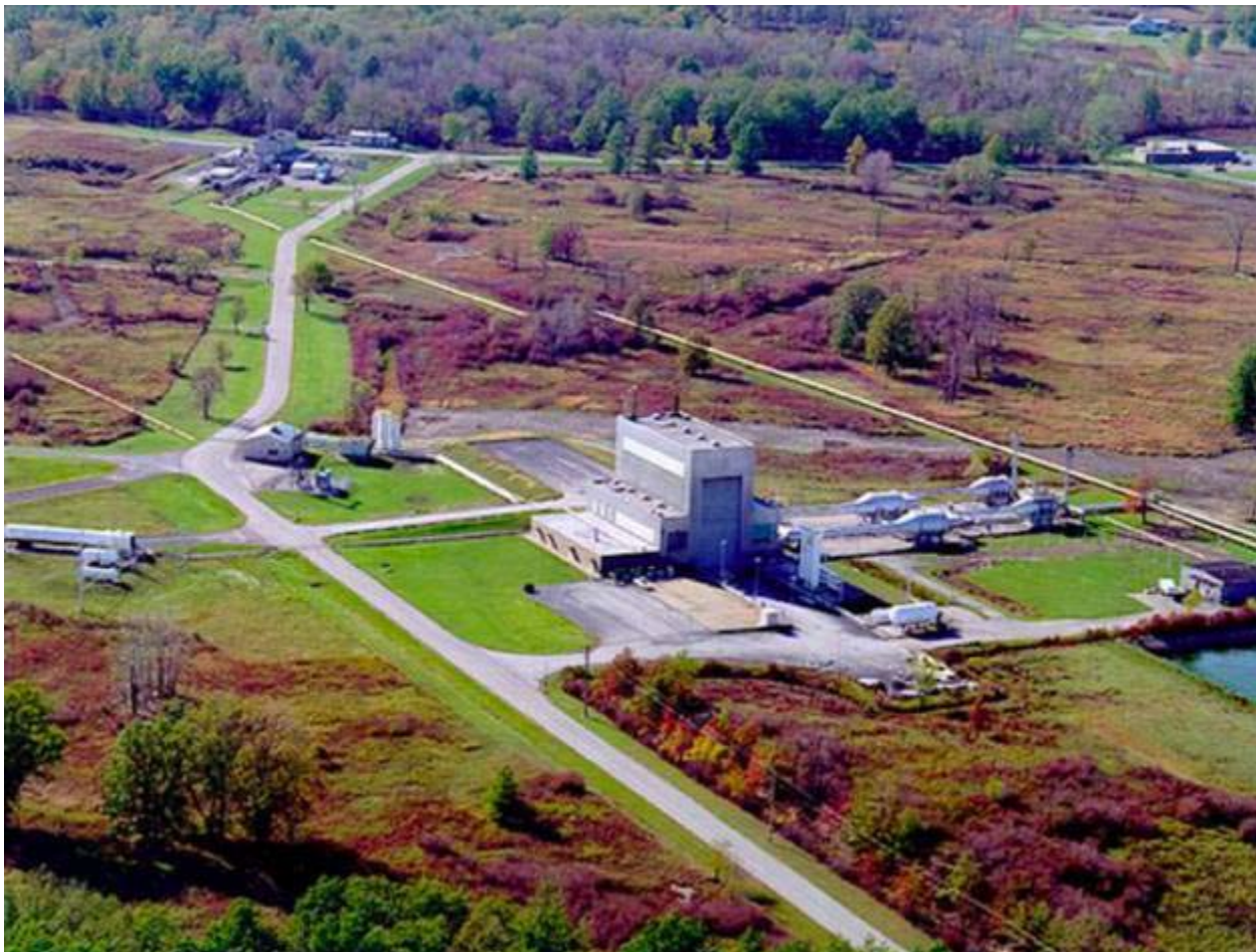
Figure 4.0-1. GRC PBS B-2 Facility Aerial View
