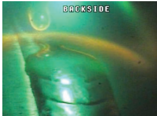
Figure 19. Segment of weld JT-08. The bead has been displaced toward the right until it has been moved almost off the joint (see transverse section fig. 21), which can be seen extending from the left edge of the bead. At this point, the joint is only being partially consumed by the weld bead.
