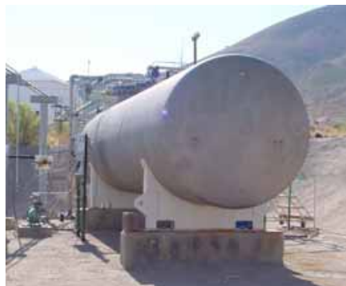
Figure 1. 300 Area Fuel Dump Tank
