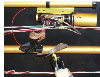
Figure 13. Air jet, modulated with a fan, causing intermittent short circuit between a wire terminal and the chassis.
