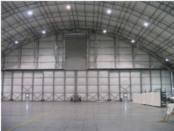
Figure 3. Space Shuttle Landing Facility (SLF) Hangar
