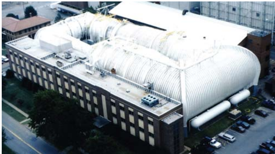
The Langley 16-Foot Transonic Dynamics Tunnel.
