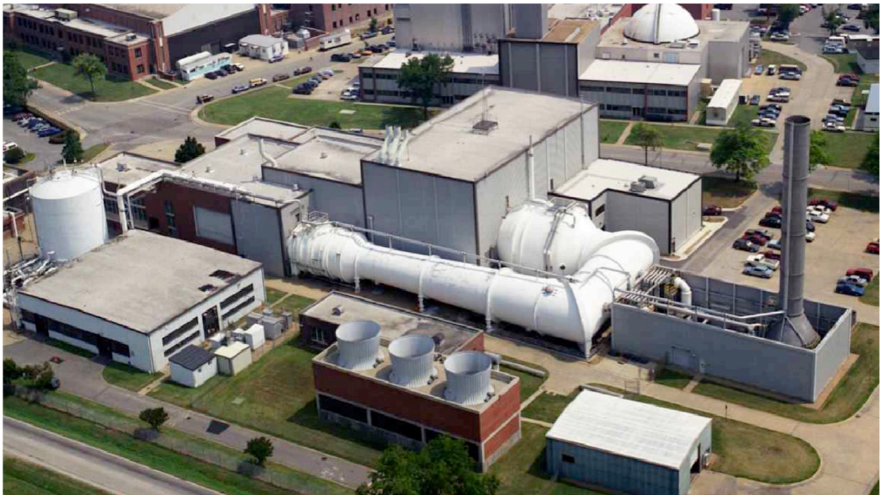
Figure 2. External view of the National Transonic Facility.
