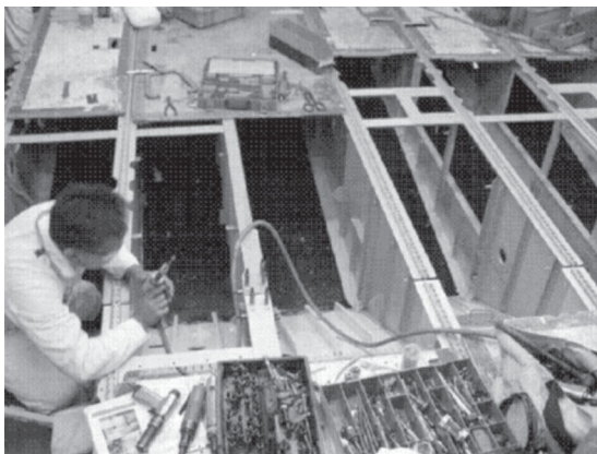
Water injection tank area during airplane construction
