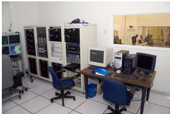
Figure 5. Photograph of BRS subsystem hardware – note view into “hotbench” area
