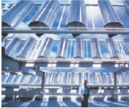
Figure 8.—A 300-kilowatt linear concentrator system (courtesy of the National Renewable Energy laboratory).
