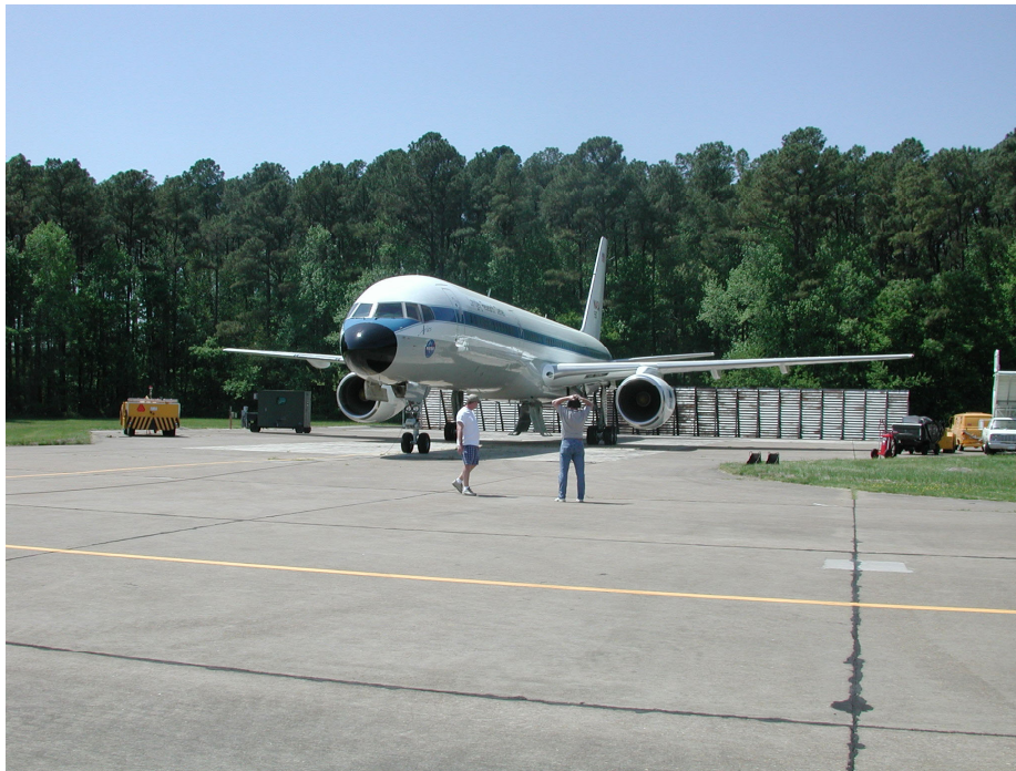
Figure 1. Photograph of the NASA Langley engine runup area showing blast fence in rear of pad with B-757 parked in front. Power and water connections are available on either side of pad.
