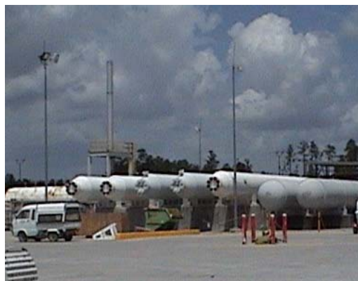
Figure 12. High pressure and high flow engine component testing is enabled by large volume “ultra-high pressure” gas supply; here the E-1 stand nitrogen supply is augmented from 3 to 5 bottles to meet the needs for the largest test articles.
