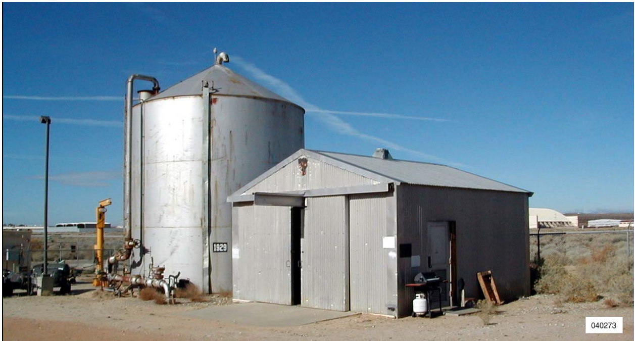
Photo courtesy NASA Dryden Flight Research Center, Edwards Air Force Base, California (Daniel S. Jones). Figure 13. The Rocket Engine Test Facility water tank and pump house.
