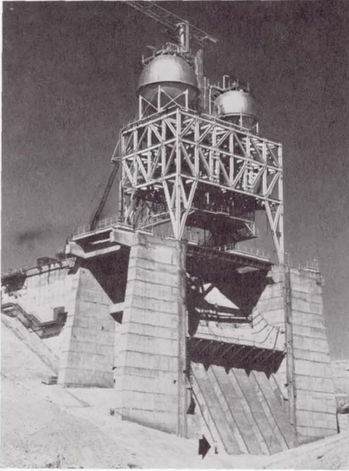
The F-1 test stand in the Mohave Desert towered 76 meters (note man at base).
