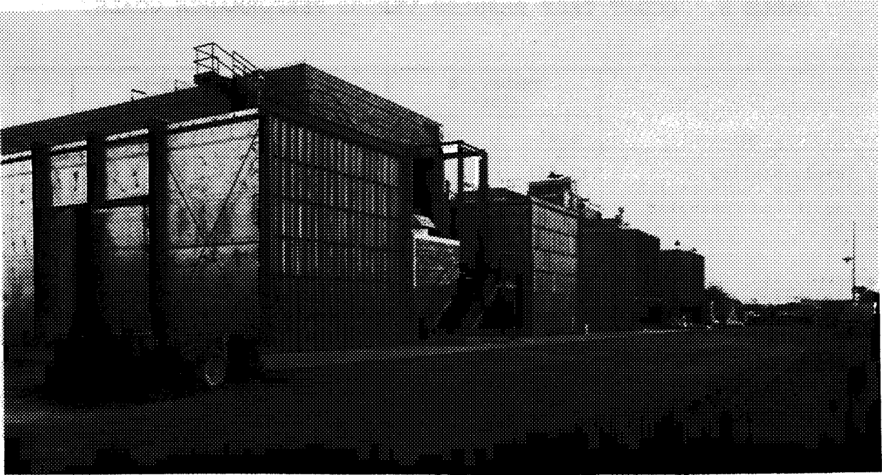
Figure 1. Development and Qualification Test Area.
