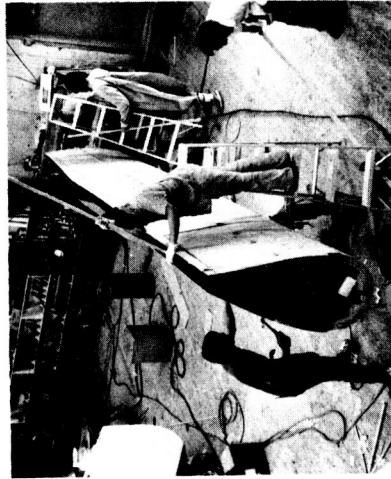
(d) Installation of opposing tail section and joining at aft tip.
