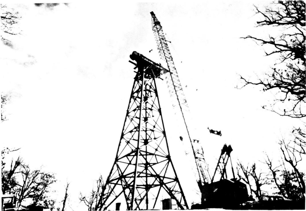
Figure 13. - WTG assembly and crane.
