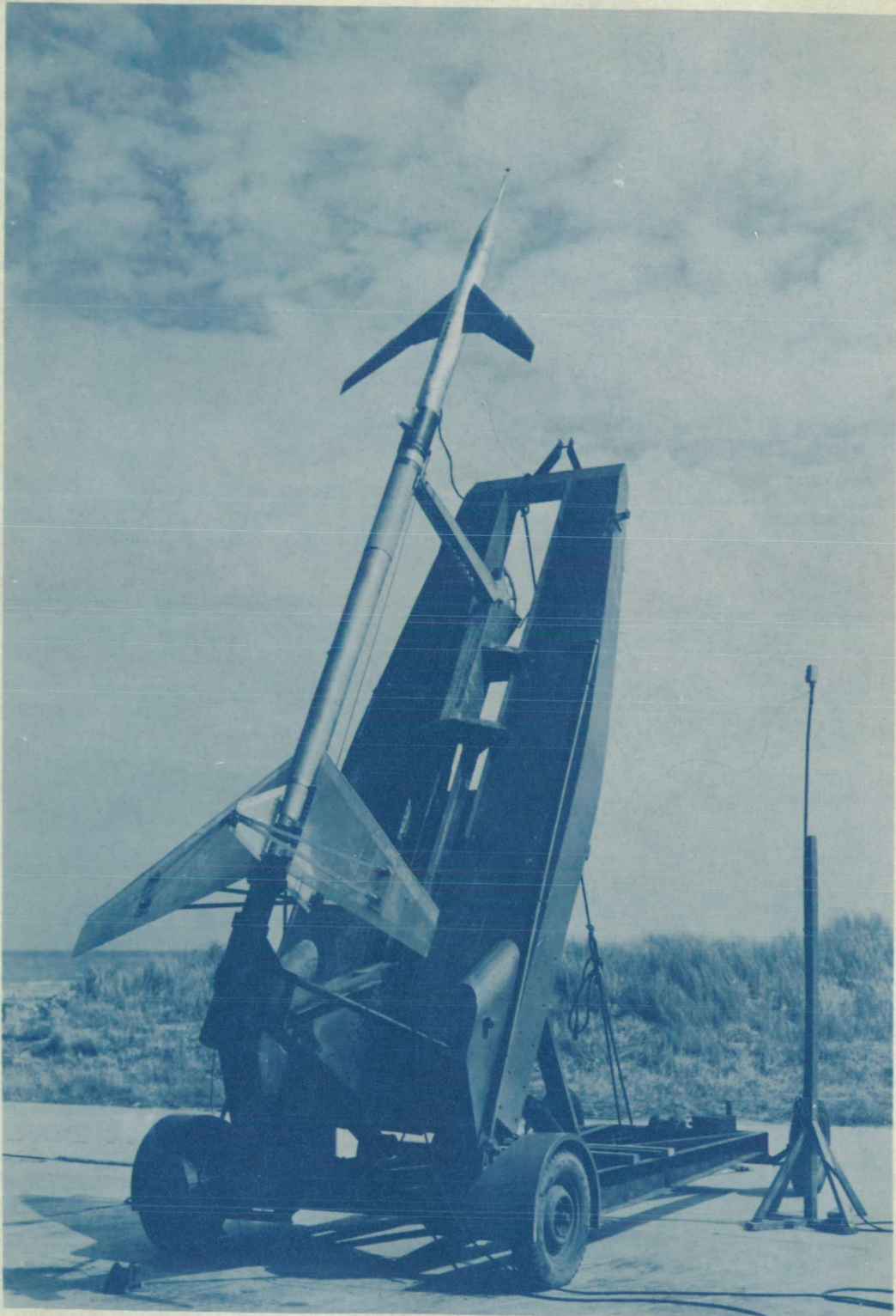
Figure 3.- Model-booster combination prior to launching.
