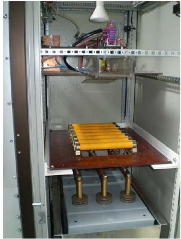
Figure 3: The replacement second harmonic anode power supply capacitors.
