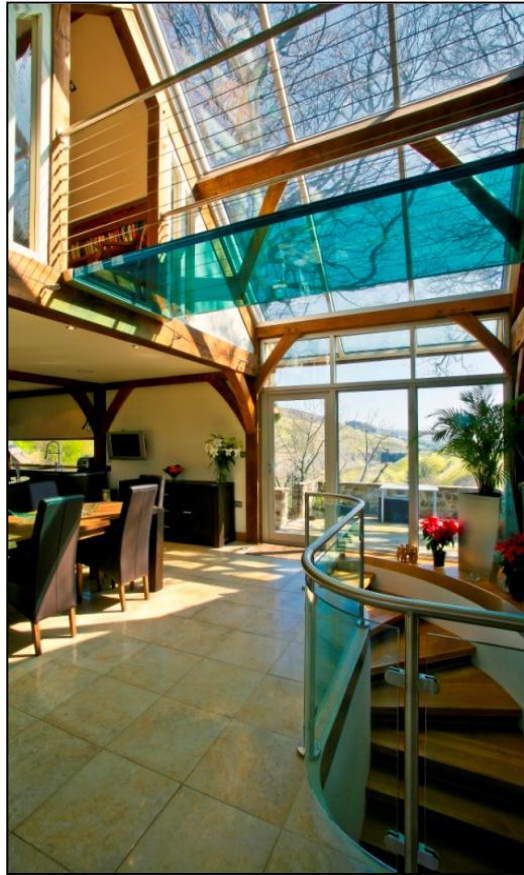
Figure 2.1 Float glass bridge and balustrade, Co. Durham, UK, 2007.
