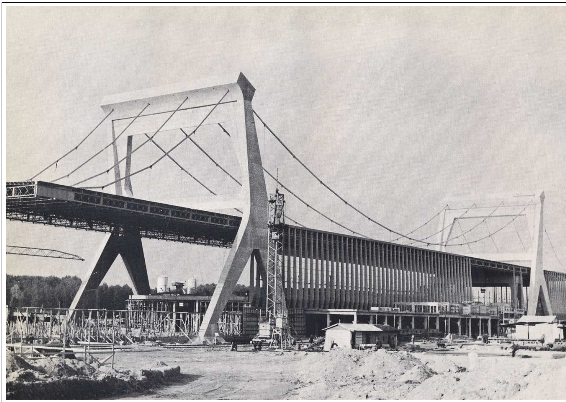
Figure 19: The Burgo Paper Mill, on site. [MAXXI]
