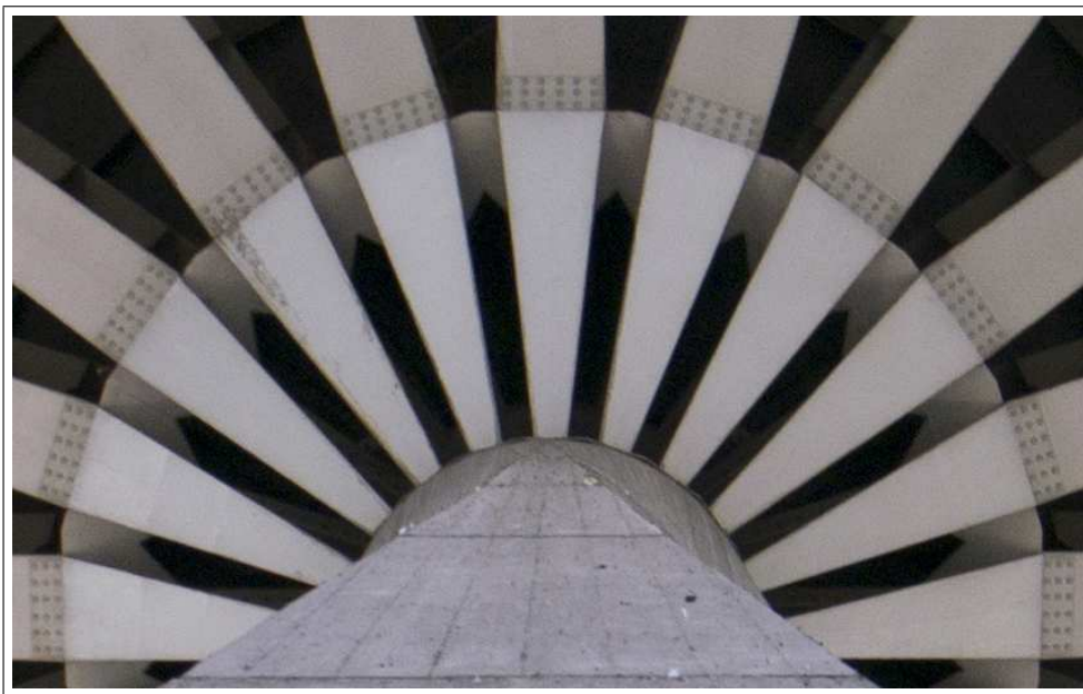
Figure 6: Detail of the bolted connection capital-beams. [MC]
