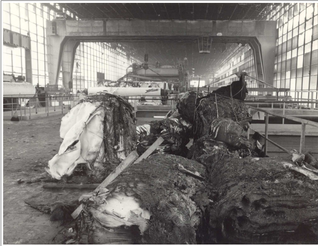
Figure 20: The Burgo Paper Mill after the fire in 1974. [BURGO]
