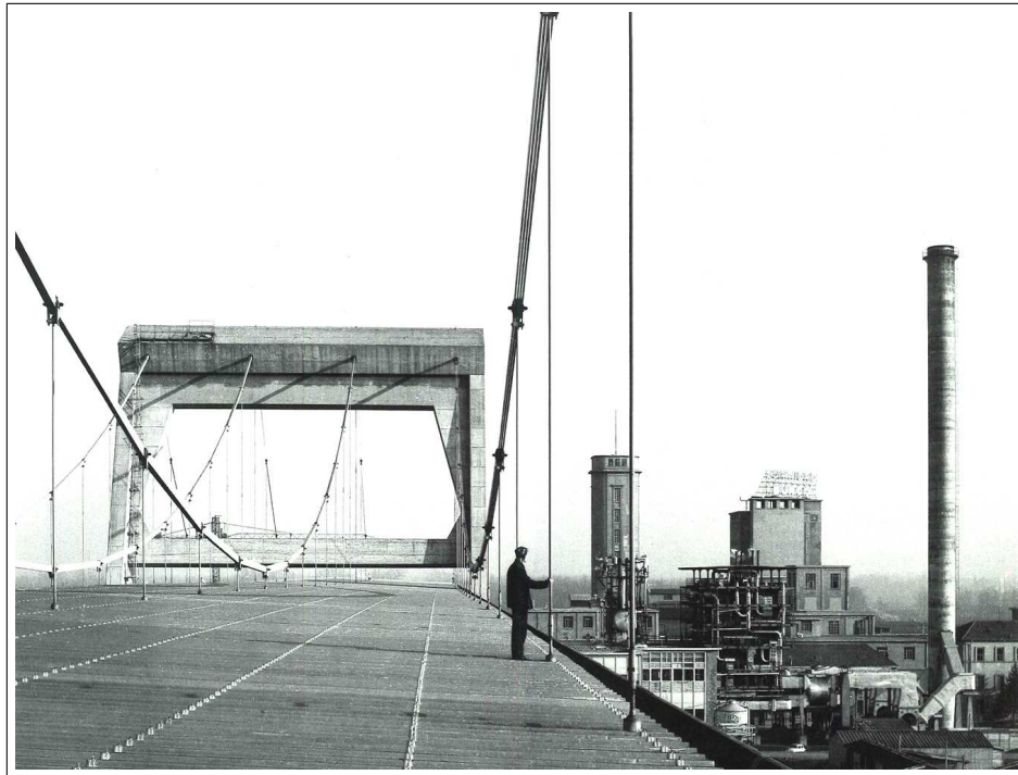
Figure 15: On the roof of the Burgo Paper Mill in 1961, Mantua. [BURGO]
