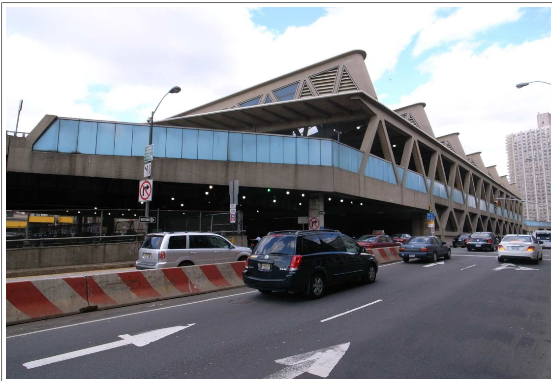
Figure 2: A view showing the two lattice beams and the structure of the roof. [MC]
