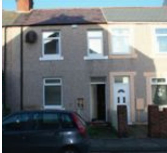
Figure 10.9. The demonstration house on Castle Terrace. Photo from Dott 07 website
