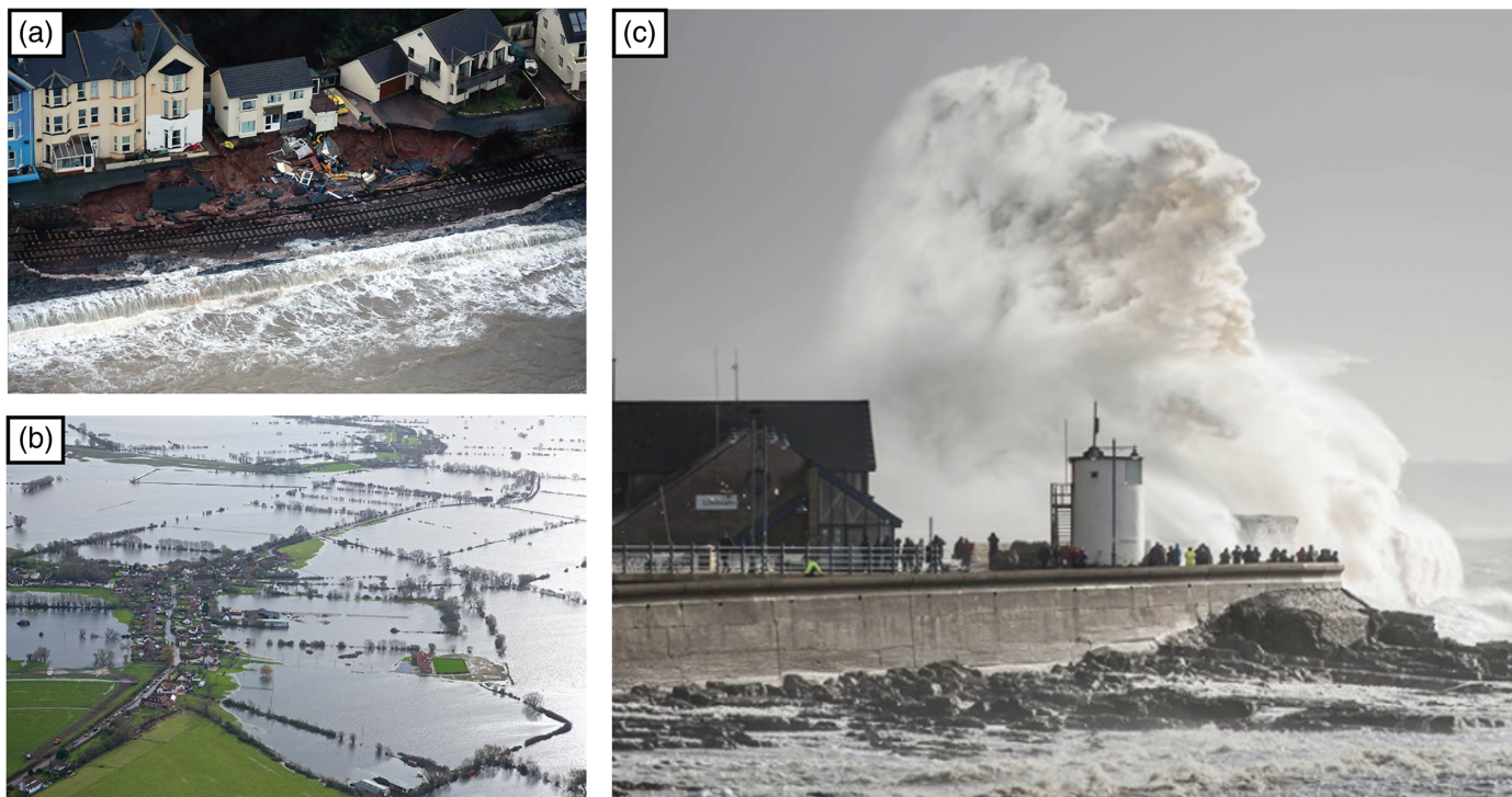
Figure 1. Images of storm impacts from DJF1314. (a) Breached sea defences and collapsed train line at Dawlish, Devon on 6 February 2014. (Source: Network Rail.) (b) The flooded Somerset Levels on 2 February 2014. (Source: Tim Pestridge.) (c) Large waves at Porthcawl, Wales on 5 February 2014. (Source: Karl Baker.)
