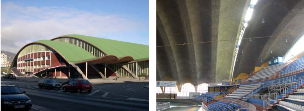
Figure 3. Exterior and interior of the Oviedo Sports Hall
